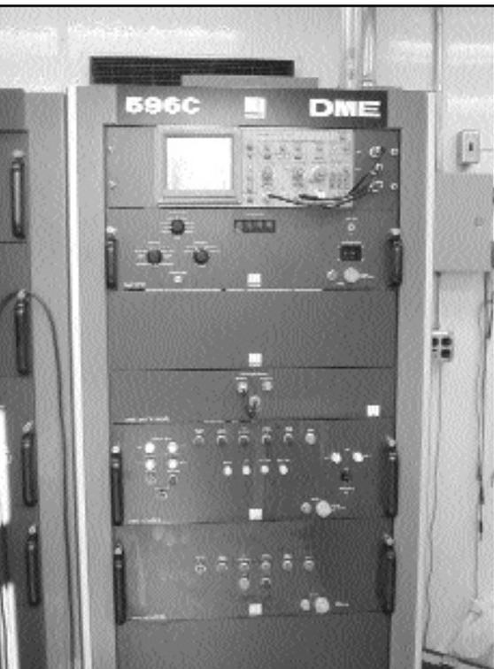
*Wilcox (Thales) DME ground station equipment rack.*
